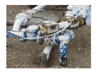
Project was to remove and repaint piping at a crude oil terminal. The existing pipe paint was flaking with pipes exhibiting surface corrosion in areas. All valves and gauges were to be masked including an aluminum cable tray. Valves to be painted red, pipe in white. The terminal was to remain in operation during the project.
